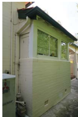
Figure 29.0, Eastern elevation showing painted brickwork and condenser for central air-conditioning. AW 2018
